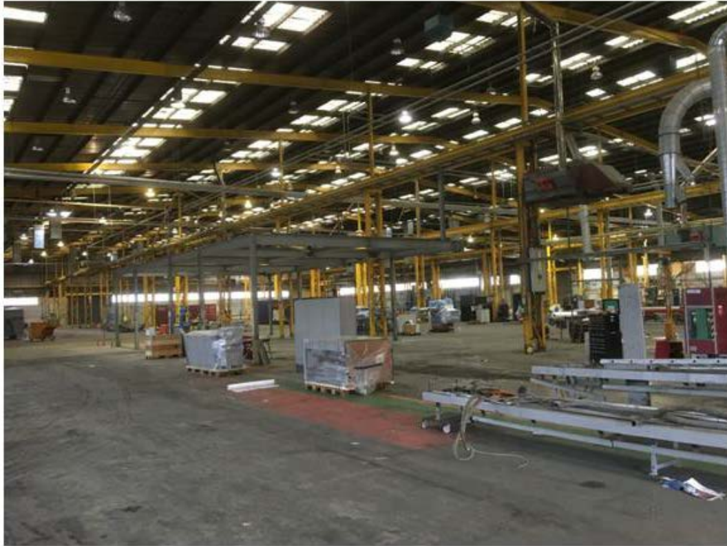
Photo 9 Steelwork left in place
